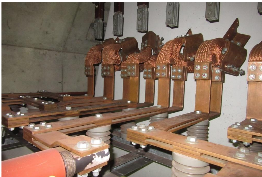
Generator bushing connections of the currently IN USE Generator in Leiden. (hence the 90 degree rotation)
