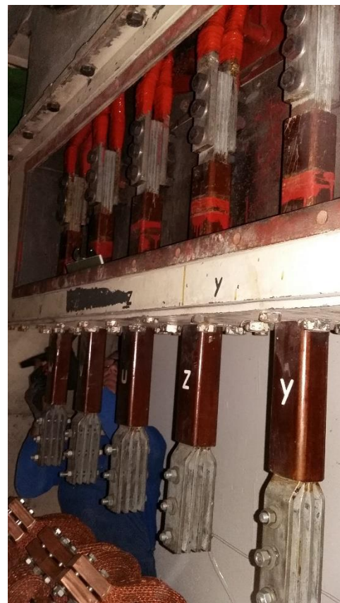
Generator bushing connections of the currently IN USE Generator in Leiden. (hence the 90 degree rotation)
