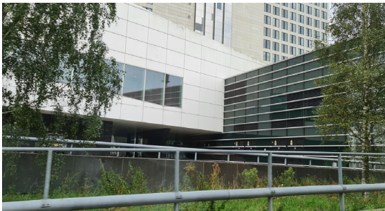
View from east side
