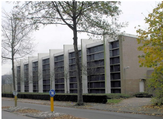
Building O (Olympia)
