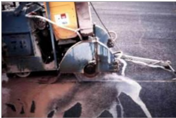
Figure 13 Cutting of the groove
