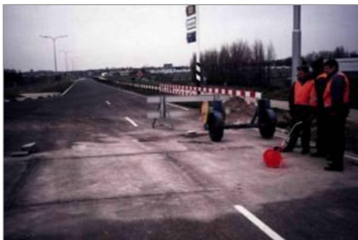
Figure 16 The grooves are cut
