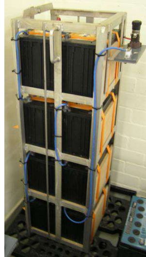
Accurek RVS verlengd met 8 accu's (racon)
