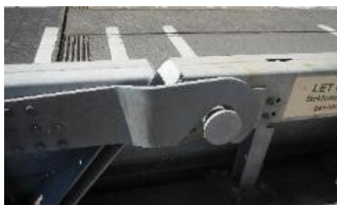
Figuur 11: Haak-nokverbinding
