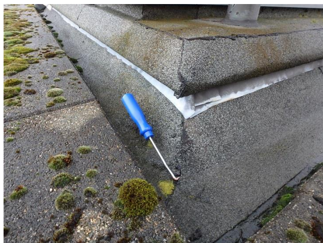
Foto 58 Onthechting overlap opstandstroken
