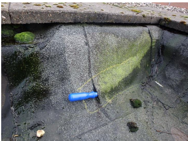
Foto 51 Onthechting overlap opstandstrook
