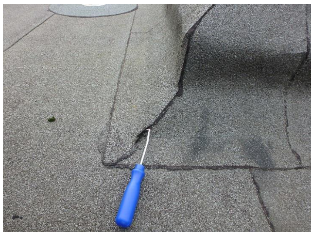
Foto 27 Onthechting overlap opstandstrook liftopbouw
