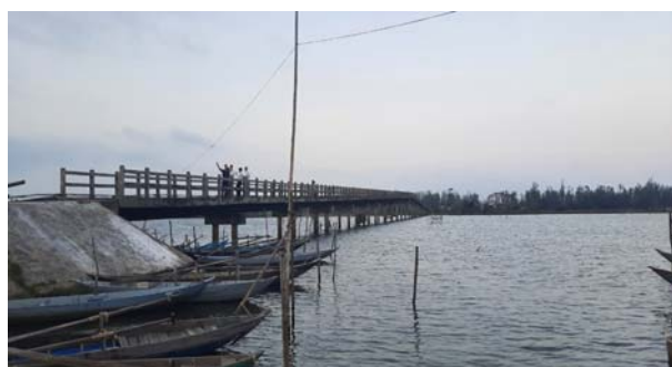
Low and narrow bridge
