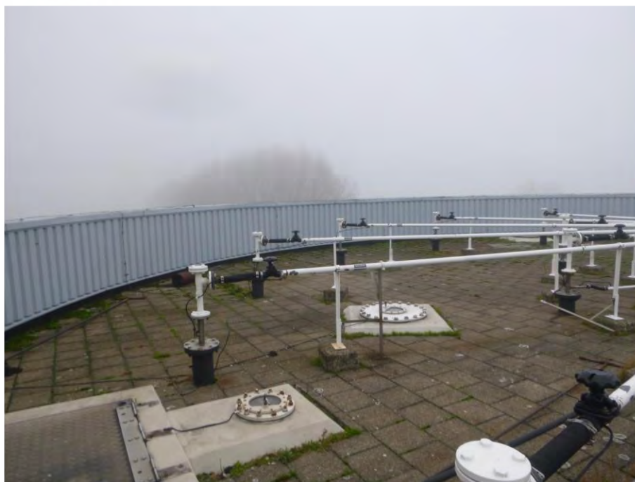
Foto F73, Coating - Slippistingstank 1 & 2
