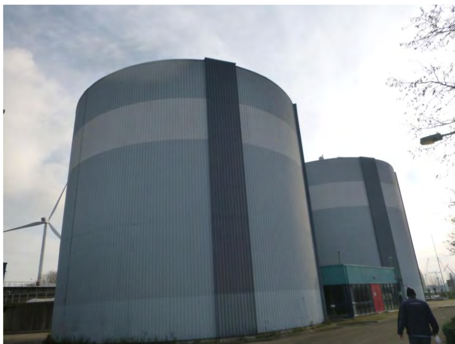
Foto F66, Coating - Slipgistingstank 1 & 2
