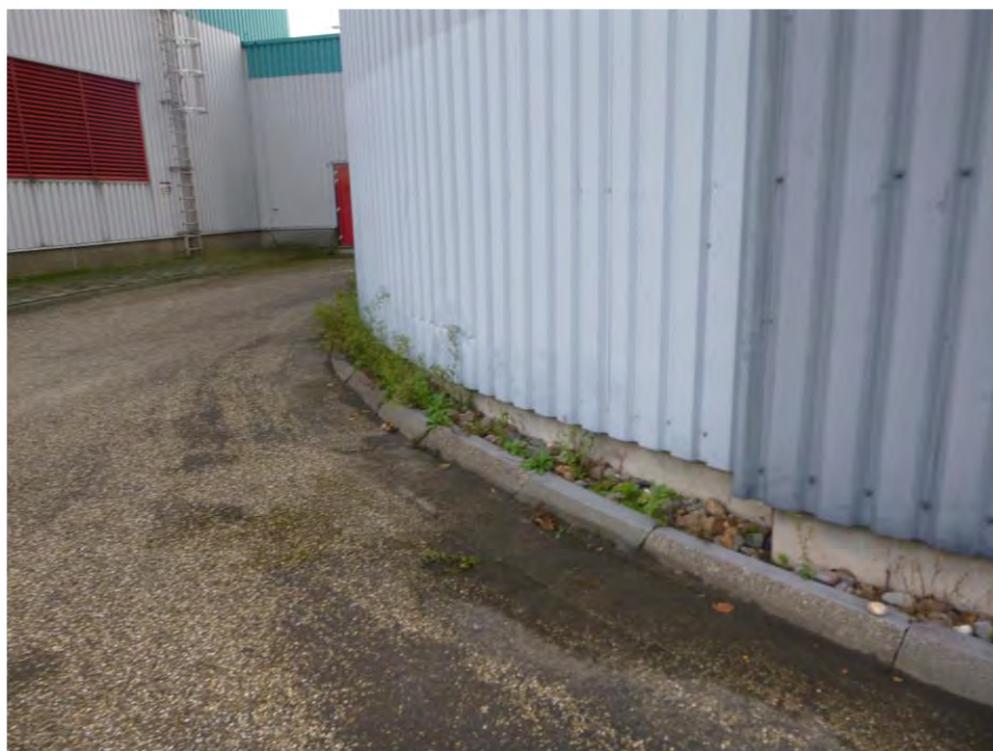
Foto F65, Beplating - Slipgistingstank 1 & 2
