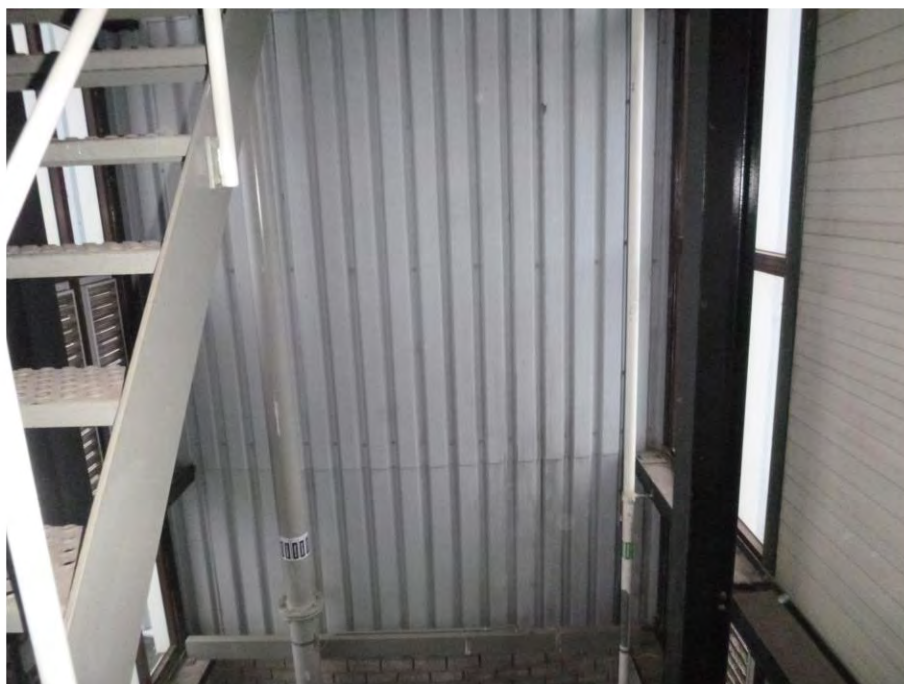
Foto F71, Coating - Slipgistingstank 1 & 2
