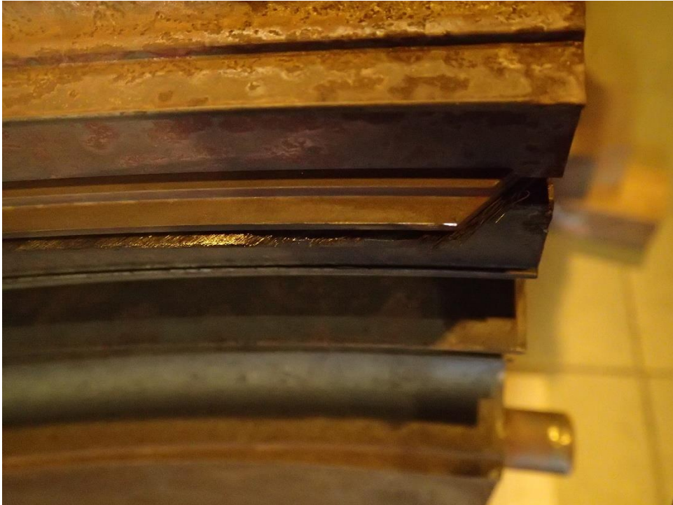
Inner Barrel Damaged Brush Seal Left Hand Side
