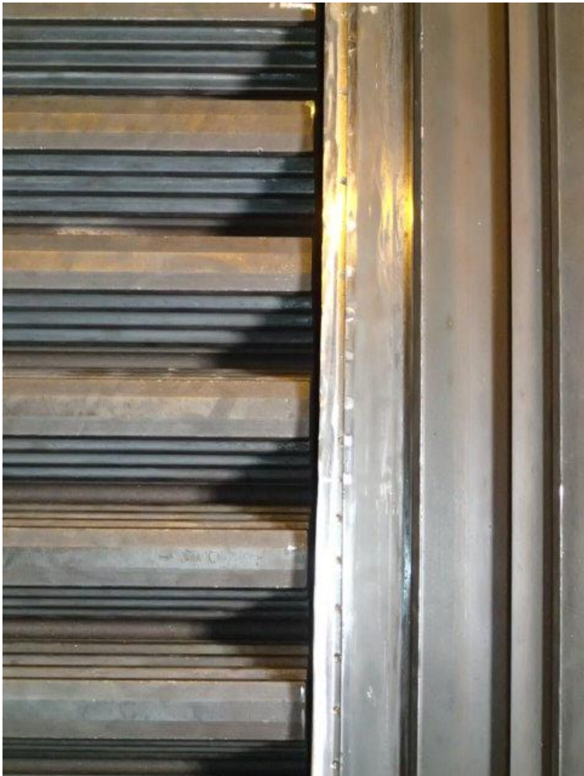
Installed new Discourager seal
