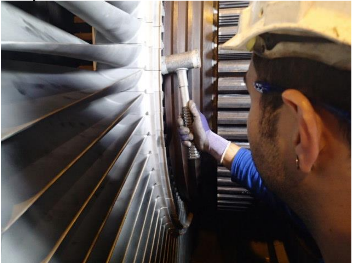
Installation of refurbished 3 rd stage Buckets
