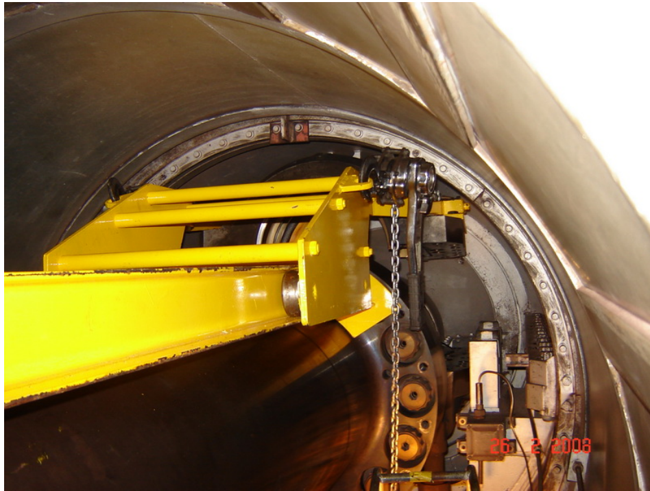
Removal of bearing cap of bearing #3
