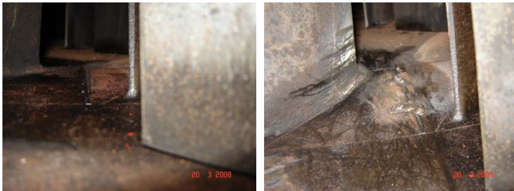
The shim before and after welding
