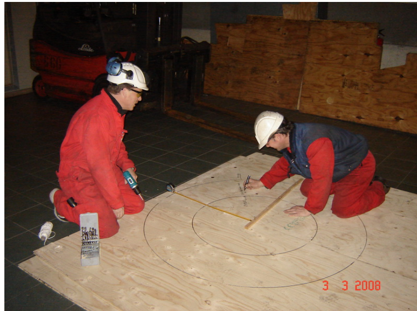
Fabrication of plywood tools for removal of bottom half of inner barrel
