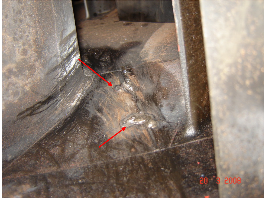
two tack welds were made to secure the protruding shim
