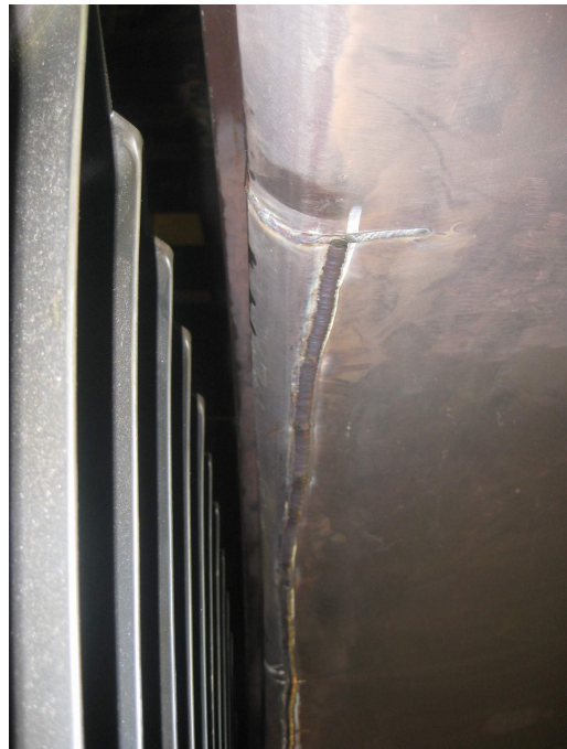
EXHAUST FLEX INTERNAL FLEX SEAL REPAIR BY EON
