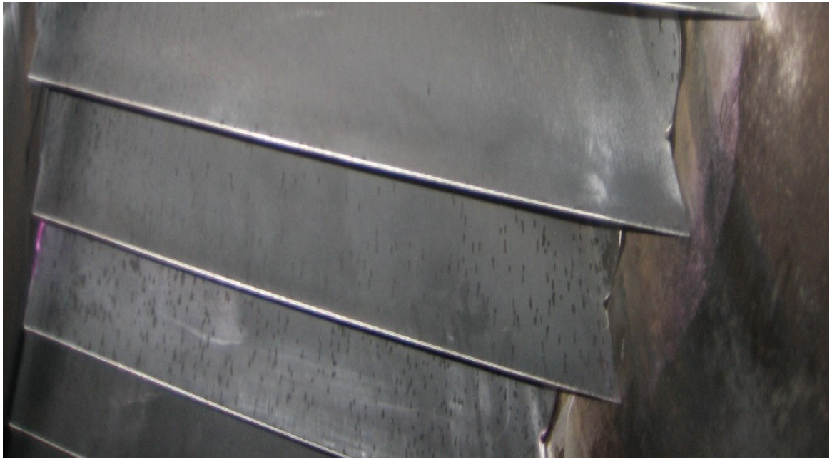
IGV GENERAL CONDITION
