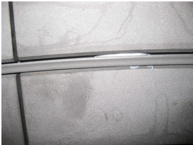
PRESSURIZED W SEAL IN PLACE
