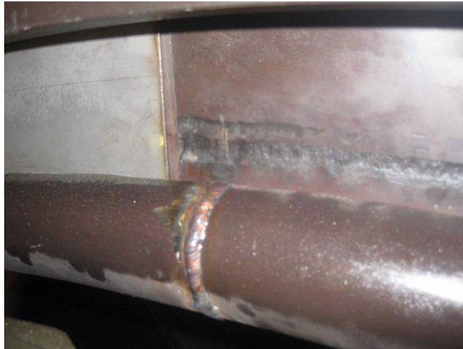
EXHAUST FLEX INTERNAL FLEX SEAL REPAIR BY EON
