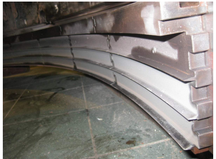
THIRD STAGE SHROUD GENERAL GOOD CONDITION
