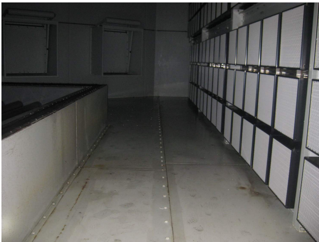
INLET PLENUM ONCE CLEANED WITH VACCUM CLEANER
