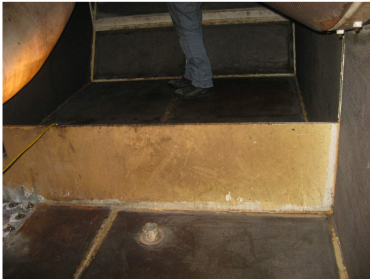
INLET PLENUM ONCE CLEANED WITH VACCUM CLEANER
