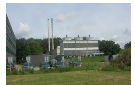
Energiecentrale in MBP
