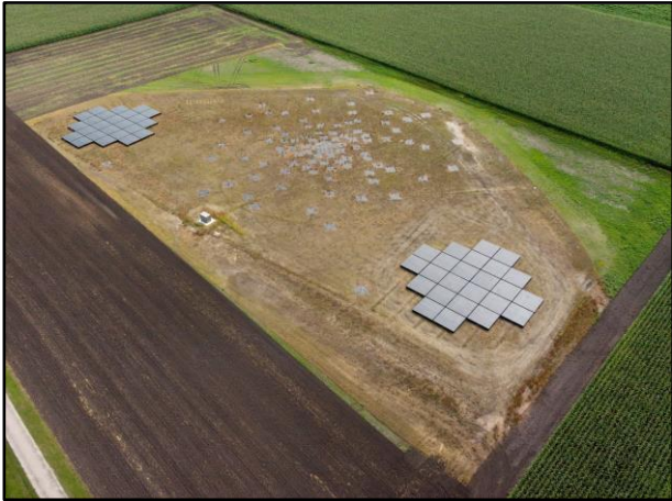
LOFAR station in de core +/- 175x100 meter
