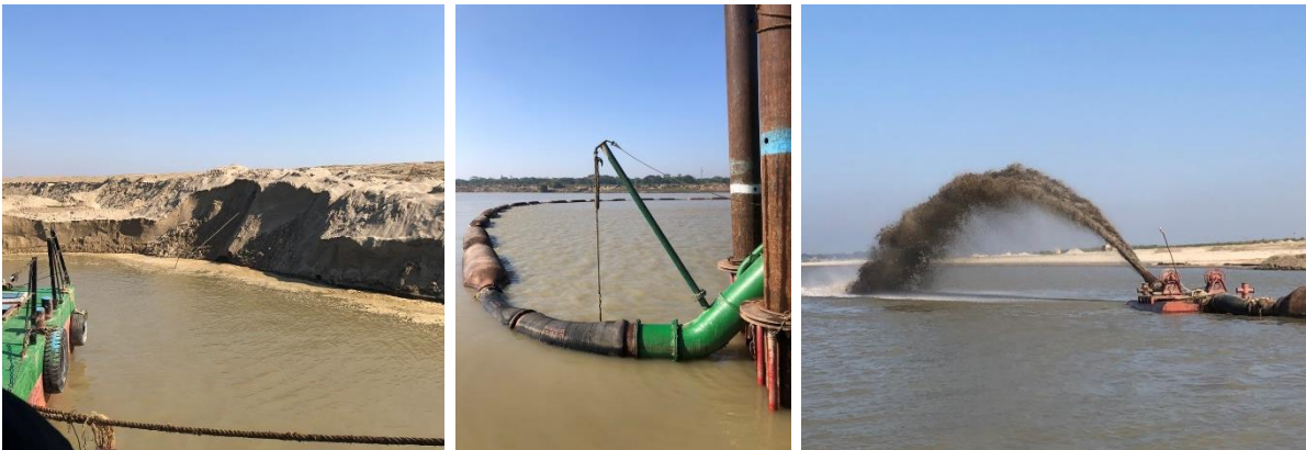
Figure 17 (left to right); formed sand point-bar across mileages 22 to 24; dredger pipeline; dredged sand/water being released back into the Ayeyarwady River.
