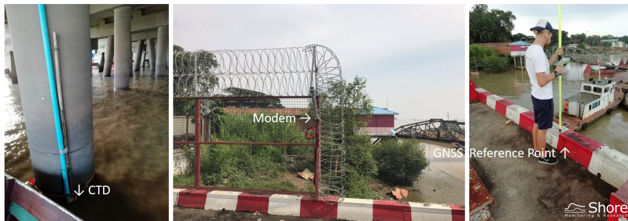
Figure C.2: Installation of Water level logger Monkey point. Left panel: location of CTD. Center panel: Location of Modem. Right panel: location of GNSS Reference Point.
