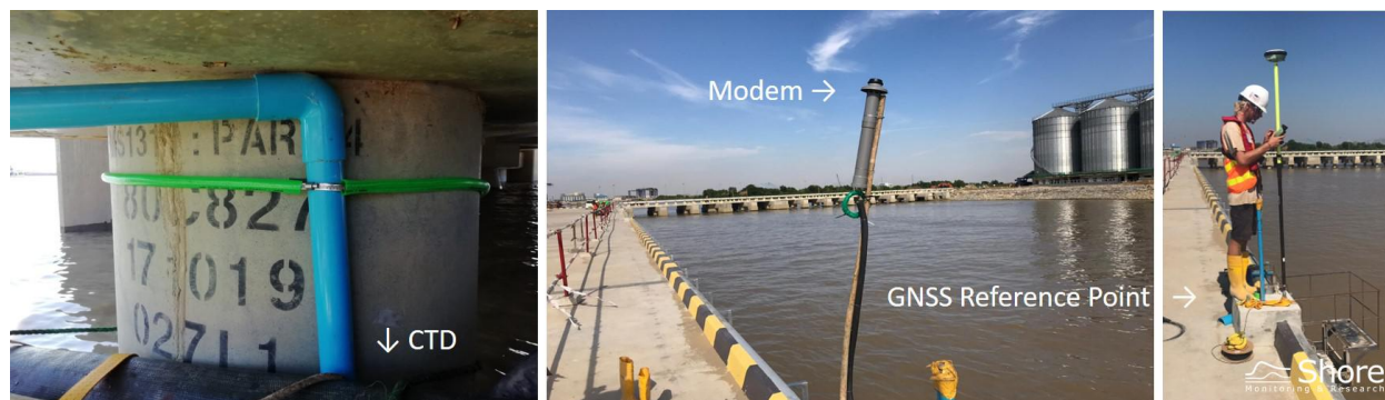
Figure C.1: Installation of Water level logger Elephant point. Left panel: location of CTD. Center panel: Location of Modem. Right panel: location of GNSS Reference Point.
