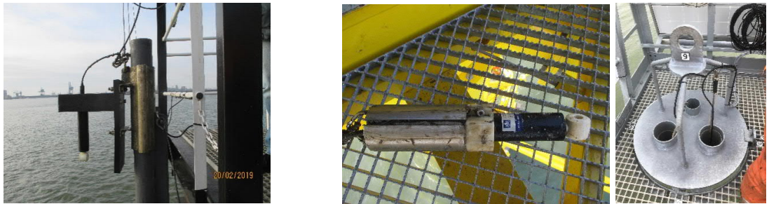
Figures 5 to 7 - Impression of fastening methods, from left to right, a block, immersion tool and tube for submerging
