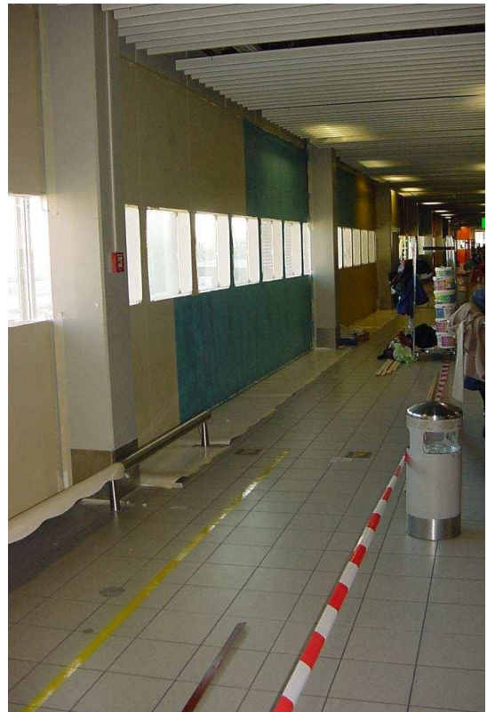
Anti-dust partitions with roof
