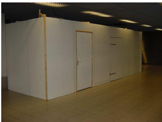
Hoardings to ceiling \pm 2.40 meters high
