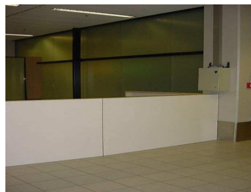
Hoardings 1.20 meter high = not desirable!
