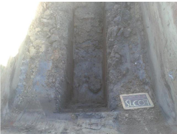
Foto 7: RE C2, sleuf SLC7
