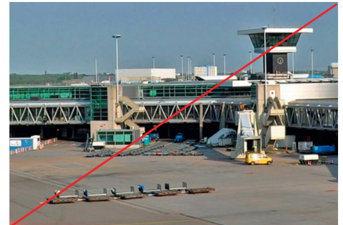
undesired layering of the façade: lack of consistency
