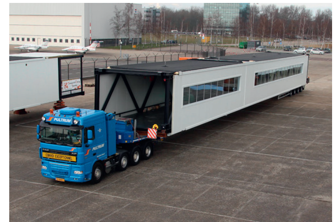
transport of a module of the temporary corridor between pier E and F
