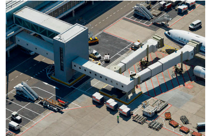
gatehouses connect the pier to the aircraft via the aviobridge
