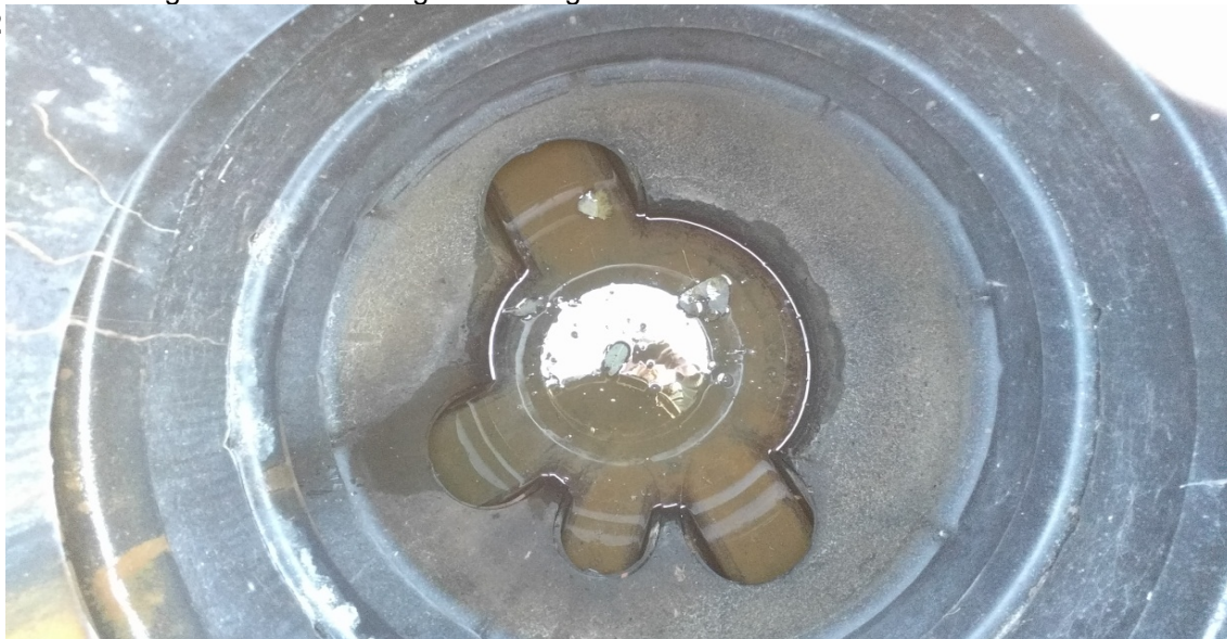
Beperkt sediment in hemelwaterdrainageput
